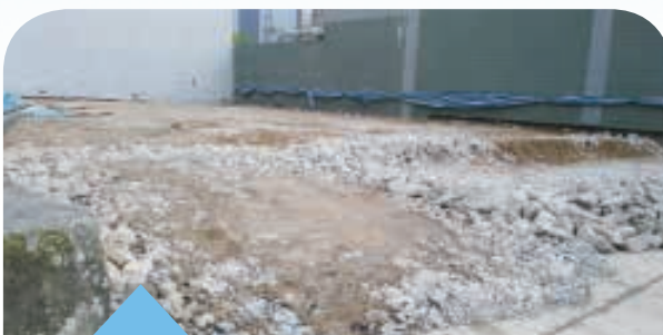
Reuse concrete for backfilling
