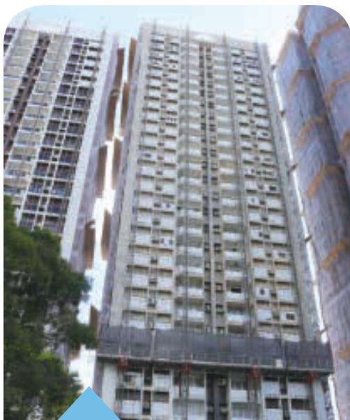
Use of Tower Working Platform for renovation works instead of bamboo scaffolding
